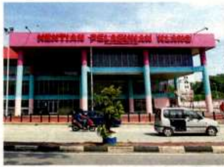
The business wing of the Port Klang Bus Station on the right is vacant.
